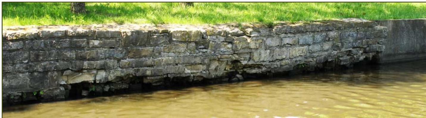
**This view of the retaining wall at the south end of the pond shows deterioration at the water line. If this wall collapses, it could affect our neighbors' properties.**
