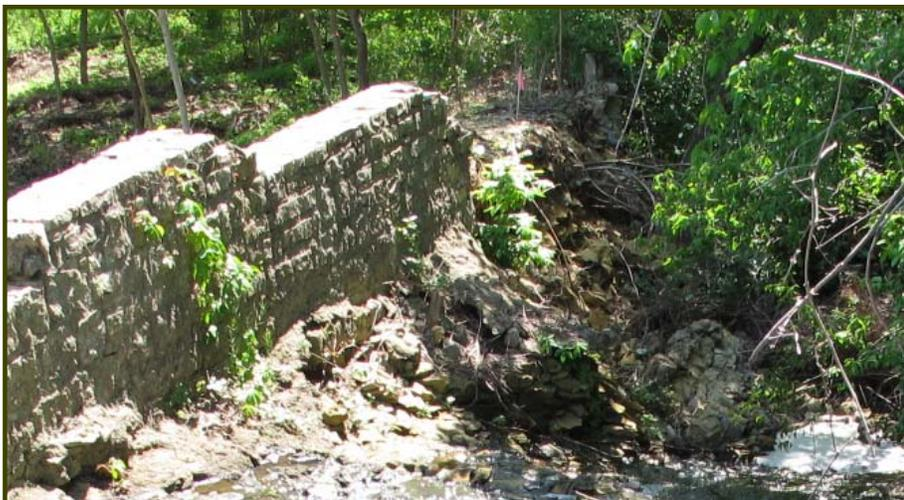
**The rock wall on the north, adjacent to the spillway, has collapsed.**
